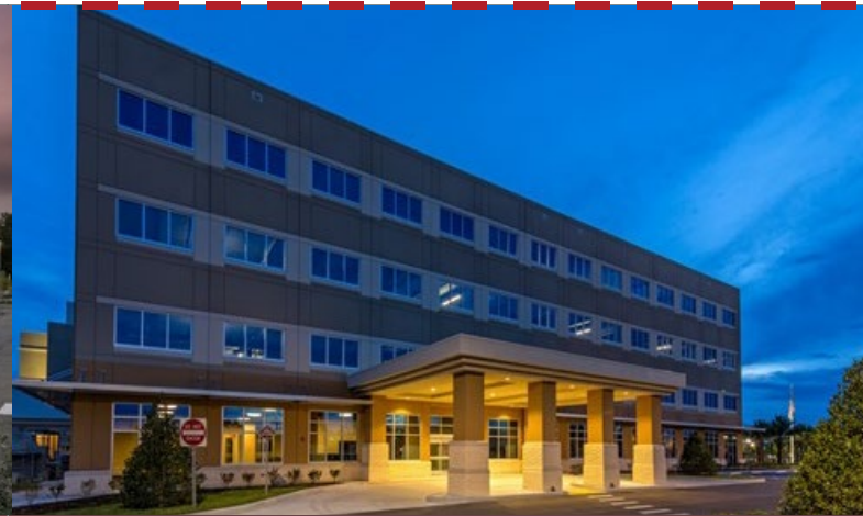
Trinity Medical Arts Building 9332 State Rd. 54, New Port Richey, FL 34655
